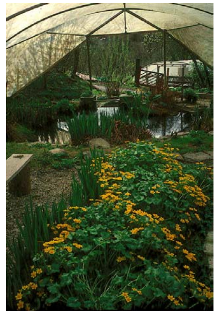
Aquatic-plant waste-water treatment facility, used also for teaching and research
