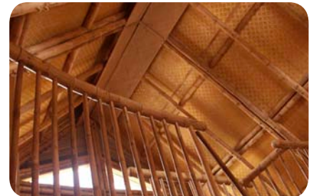
Vaulted ceilings with bamboo trusses
