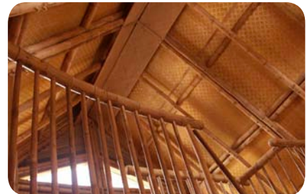
Vaulted ceilings with bamboo trusses
