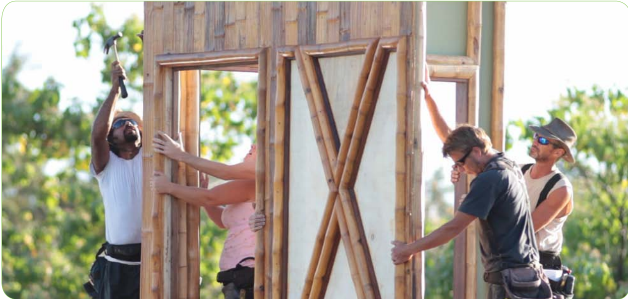
Contractors assembling the Bamboo Living exterior wall panels.
