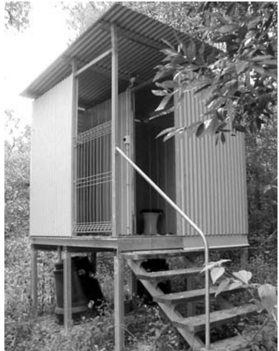
AN OFF-THE-SHELF COMPOSTING TOILET (ABOVE) AND AN AEROBIC WASTEWATER TREATMENT SYSTEM (BELOW)
