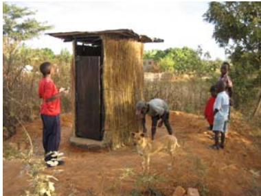
Simple grass spiral superstructures can be upgraded step by step Vent pipes can also be fitted to simple grass structures
