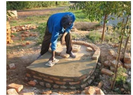
The curved extension to the 1.2m slab is built up in bricks to the height of the slab 85cm away from the slab. The brickwork also built up across the entrance as shown.
