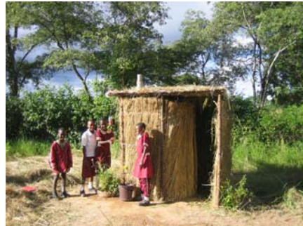
Simple grass spiral superstructures can be upgraded step by step Vent pipes can also be fitted to simple grass structures
