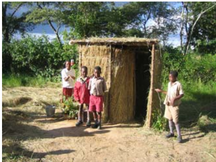
Simple grass spiral superstructures can be upgraded step by step Vent pipes can also be fitted to simple grass structures
