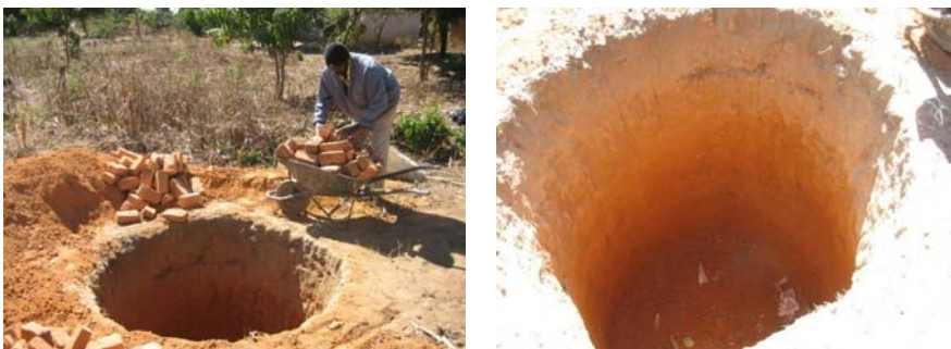
The pit is dug 1.7m wide and 2m deep. Walls are straight and bottom flat
