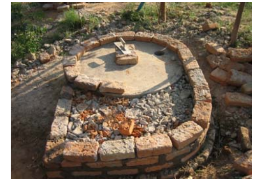
The curved extension to the 1.2m slab is built up in bricks to the height of the slab 85cm away from the slab. The brickwork also built up across the entrance as shown.
