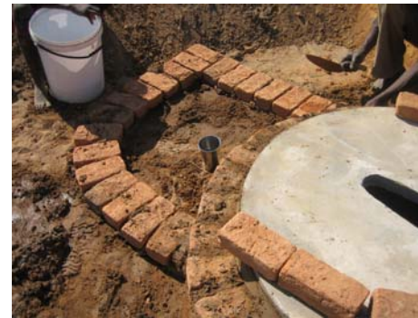
The curved extension to the 1.2m slab is built up in bricks to the height of the slab 85cm away from the slab. The brickwork also built up across the entrance as shown.
