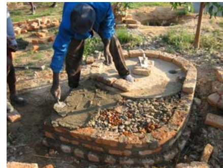
The curved extension to the 1.2m slab is built up in bricks to the height of the slab 85cm away from the slab. The brickwork also built up across the entrance as shown.
