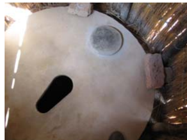
Simple grass spiral superstructures can be upgraded step by step Vent pipes can also be fitted to simple grass structures
