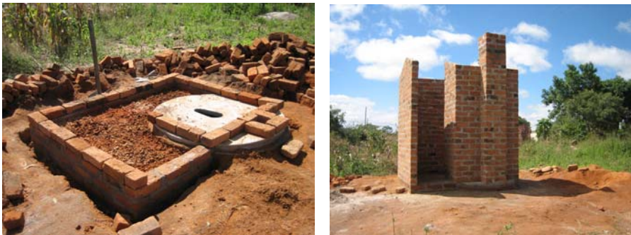
Selected photos of construction
