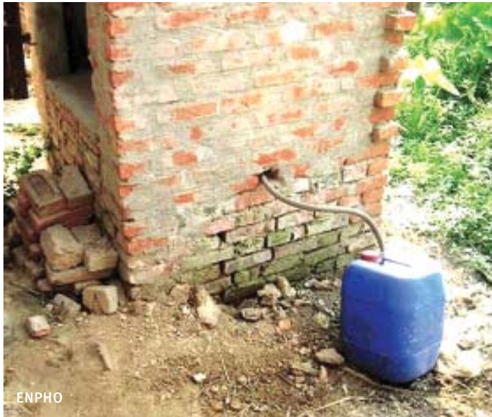
Photo 4.4: Urine collection tank
