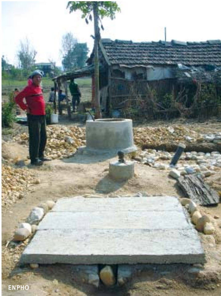
Photo 2.4: Newly constructed biogas plant with inlet for toilet
