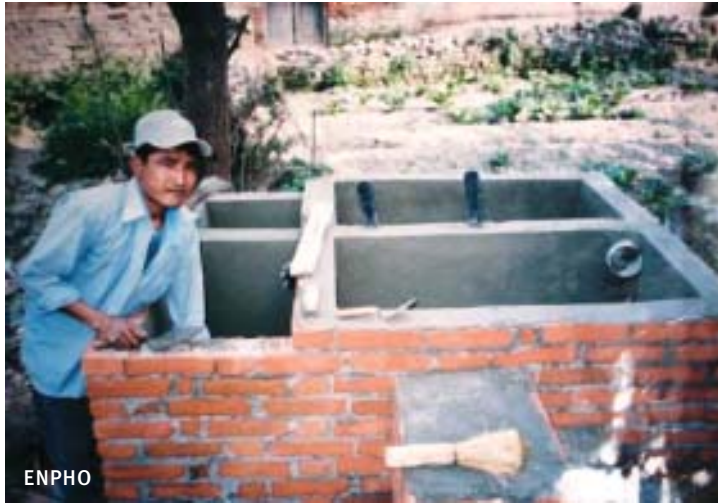
ENPHO Photo 3.2: DVUD toilet under construction
