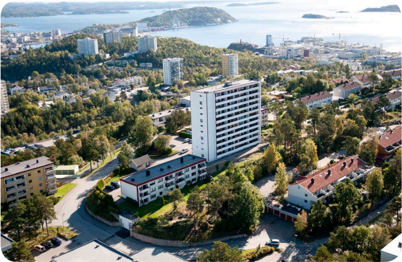
High-rised, low-rised and terraced houses from the Co-operative Housing Association Sorlandet BBL, Kristiansand (Kjell Inge Soreide)
