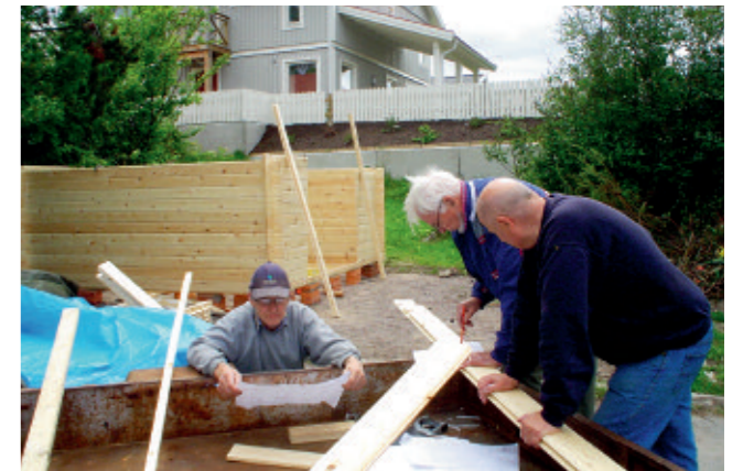
Building construction, Tersen, Falun.
