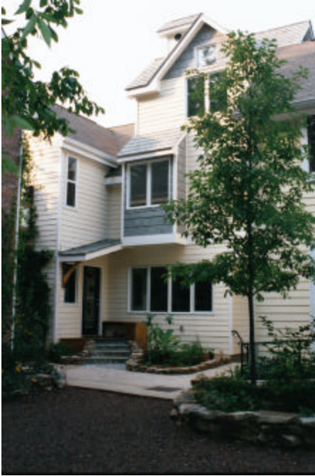
Figure B-24. View from the west courtyard to south house row. Forms and materials are similar for the common house (to the right) and the units, however, buildings are articulated to provide visual variety and human scale.
