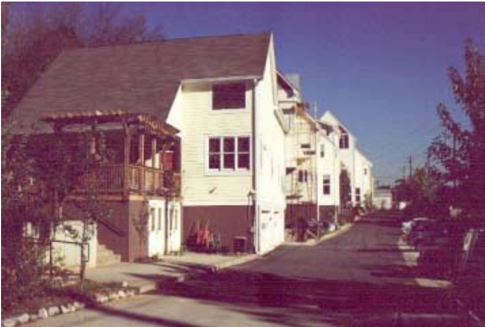
Figure B-14. Parking lot. The buildings form a barrier toward the parking lot to detach the community from undesirable environs. The stairs and handicap access ramp to the left are needed to negotiate a 2.7 m (9-foot) level difference from the parking lot to the commons. Below the common house porch is garden equipment storage.
