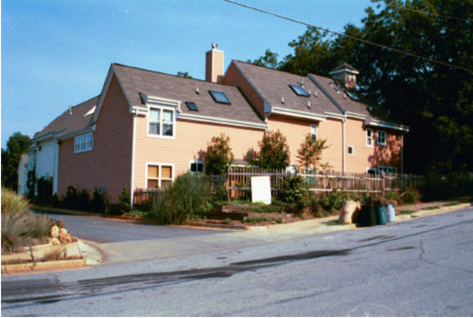
Figure B-17. Monterrey Street façade. The cohousing property features an open entrance to the parking lot and only a wooden fence along this border. Backyards are given minimum maintenance presumably to make them less inviting to strangers.
