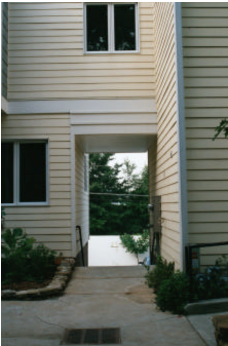
Figure B- 25. Entrance from the parking lot—Gateway 2—between the common house and the south house row. The unit closest to the common house was expanded by building over the air space between the buildings; as a result the existing passage was closed overhead, defining a third portal.
