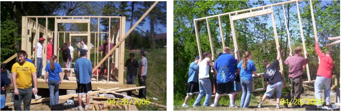
Figure 5: Some more pictures during construction
