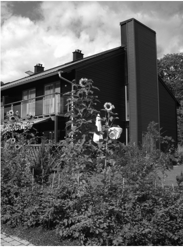
Picture 7.2 Low energy, passive, energy houses in Lindås outside Göteborg. Swedish demonstration project from 2001. In these houses the traditional heating system has been replaced by a heat exchanger in combination with an exceptionally well insulated construction. For more information see http://www.formas.se/docs/Bokhandel/houses_without_heating_systems.pdf (Photo Liane Thuvander)
