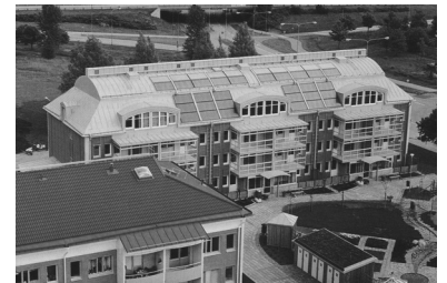
Photo 8.2 Ekoporten, Norrköping, Sweden. Architect FFNS. Photo from brochure “Ekoporten – framtidens boende i kretsloppshus” Hyresbostäder Norrköping
