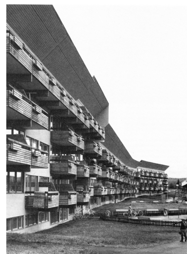
Photo 7.7 Sub arctic houses, Svappavara, Kiruna, Sweden. The project has social and climatic ambitions. Architect Ralph Erskine, built 1963. (Photo Richard Einzig, In Egelius, Mats (1988) Ralph Erskine, arkitekt . Stockholm: Byggeförlaget p. 98)
