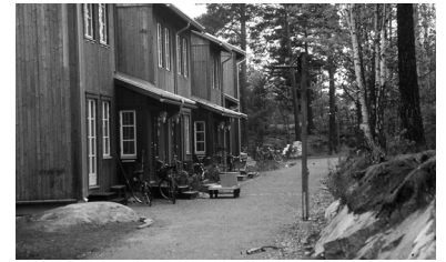
Photo 8.1 Understeshöjden, Stockholm, Sweden. Architect Bengt Bilén (Photo Michael Edén)
