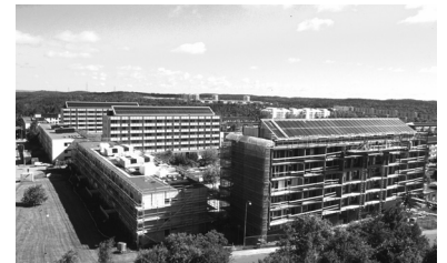
Photo 8.3 ‘Solar multi-family blocks’, Gårdsten, Göteborg, Sweden. Architect Christer Nordström Arkitektkontor.
